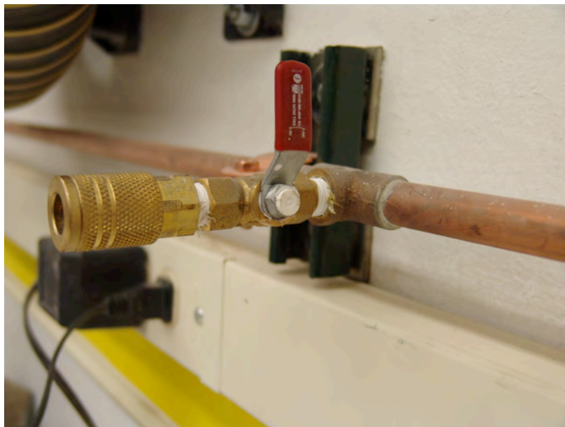
Figure 5. This image shows a work station air valve in the off position.
